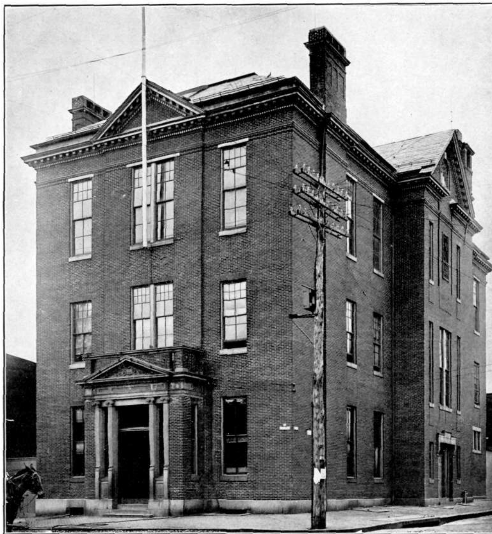
SOUTHWESTERN POLICE STATION
