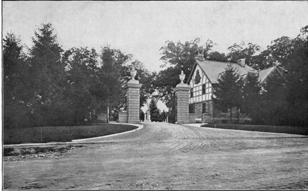
MAIN ENTRANCE LOUDON PARK CEMETERY—FREDERICK ROAD.
