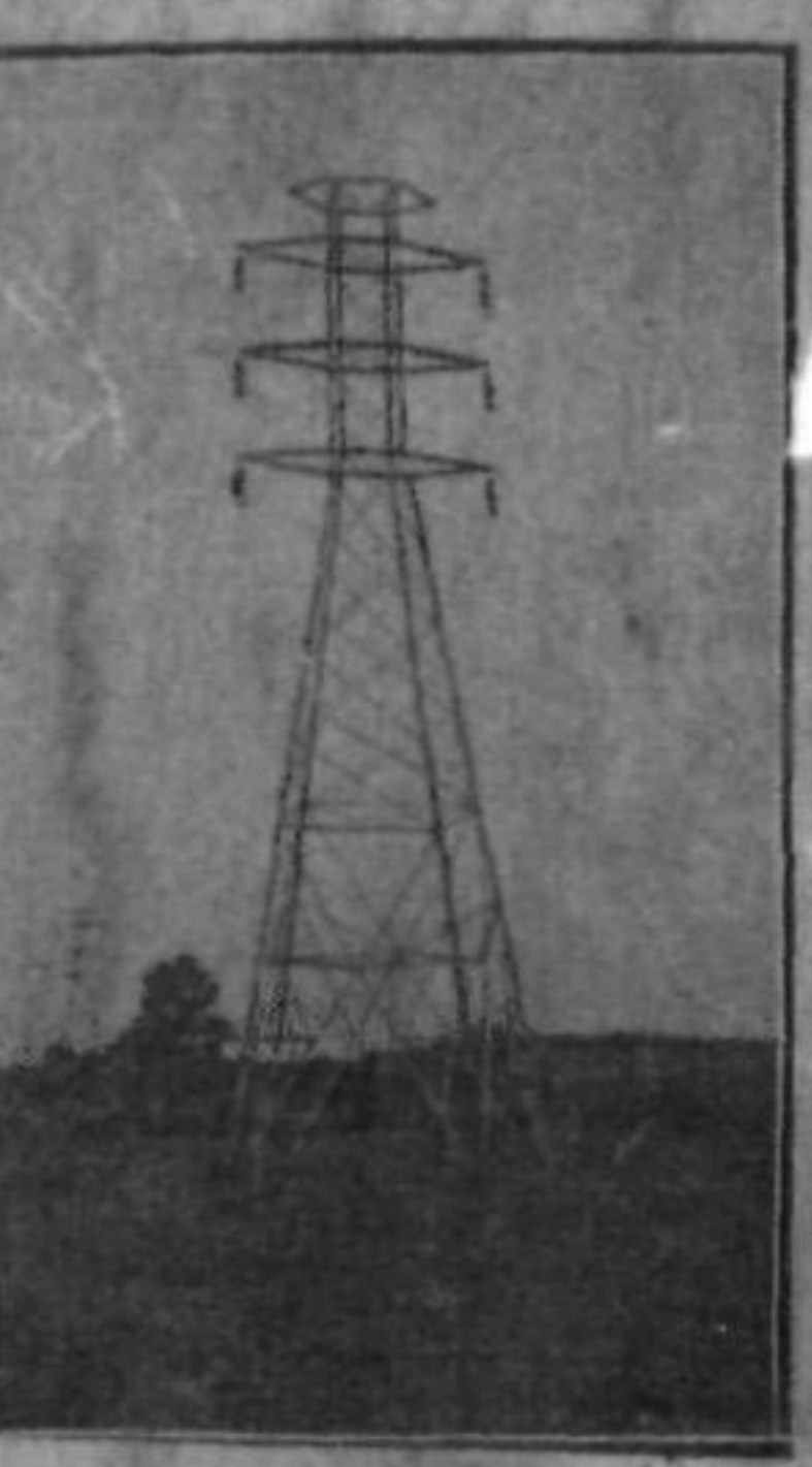
One of Transmission Towers on Line to Baltimore
