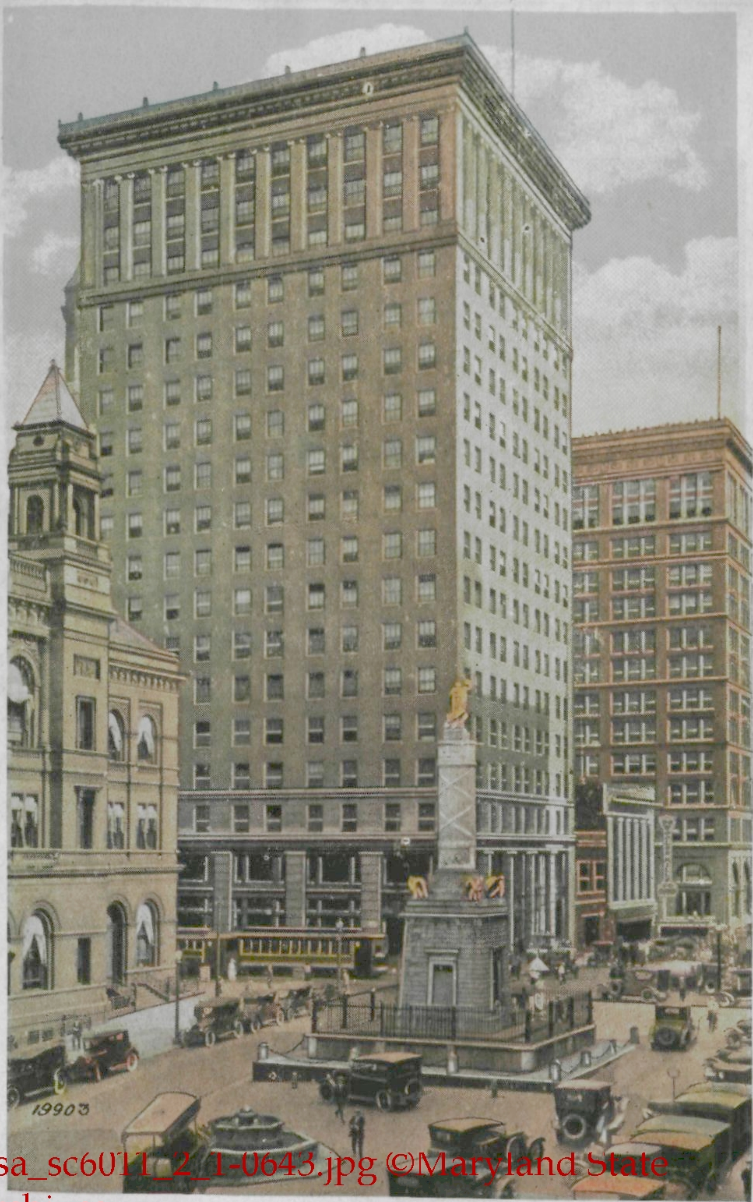
Munsey Building, Baltimore, Md.
