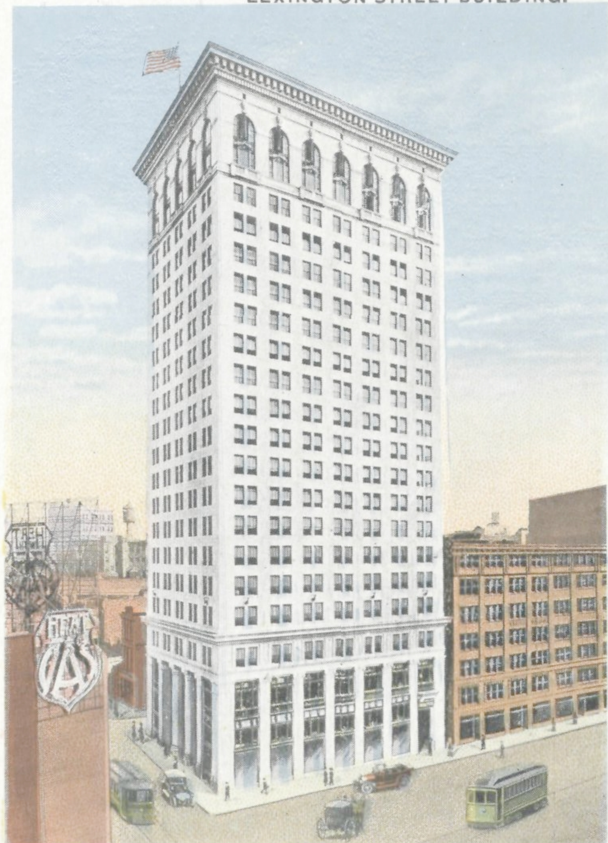
LEXINGTON STREET BUILDING.
