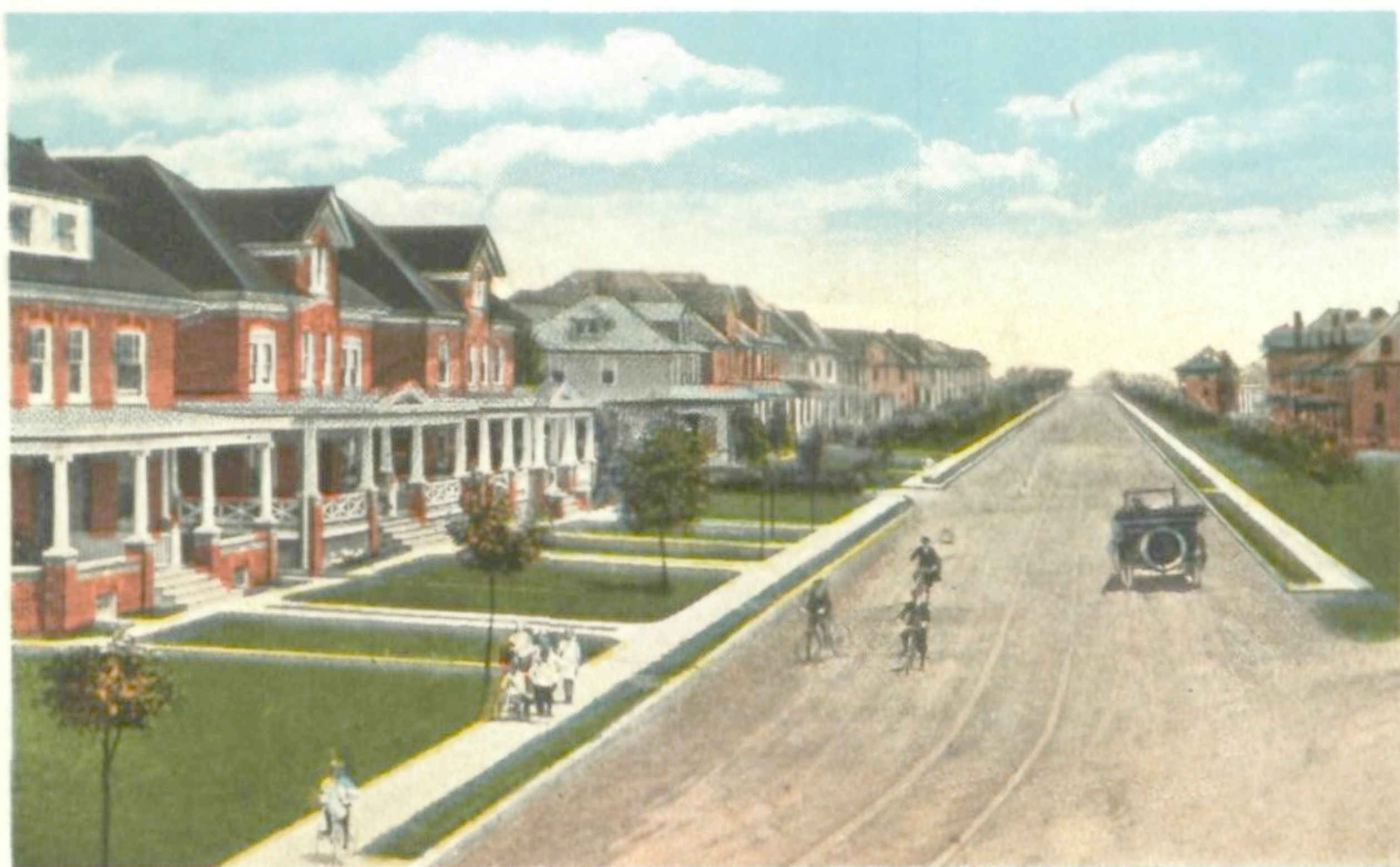
HAMILTON BOULEVARD, LOOKING NORTH.
