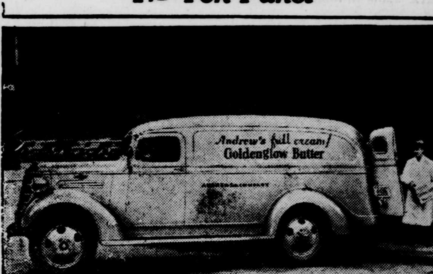
The streamlined design, all-steel top, and beaver-tail rear of the new 1938 Chevrolet 1½-ton Panel truck make it outstanding among the larger trucks. The load space is 112¼ inches long, 57¼ inches wide, and 44½ inches high. This model is built on a 131½-inch wheelbase chassis.
