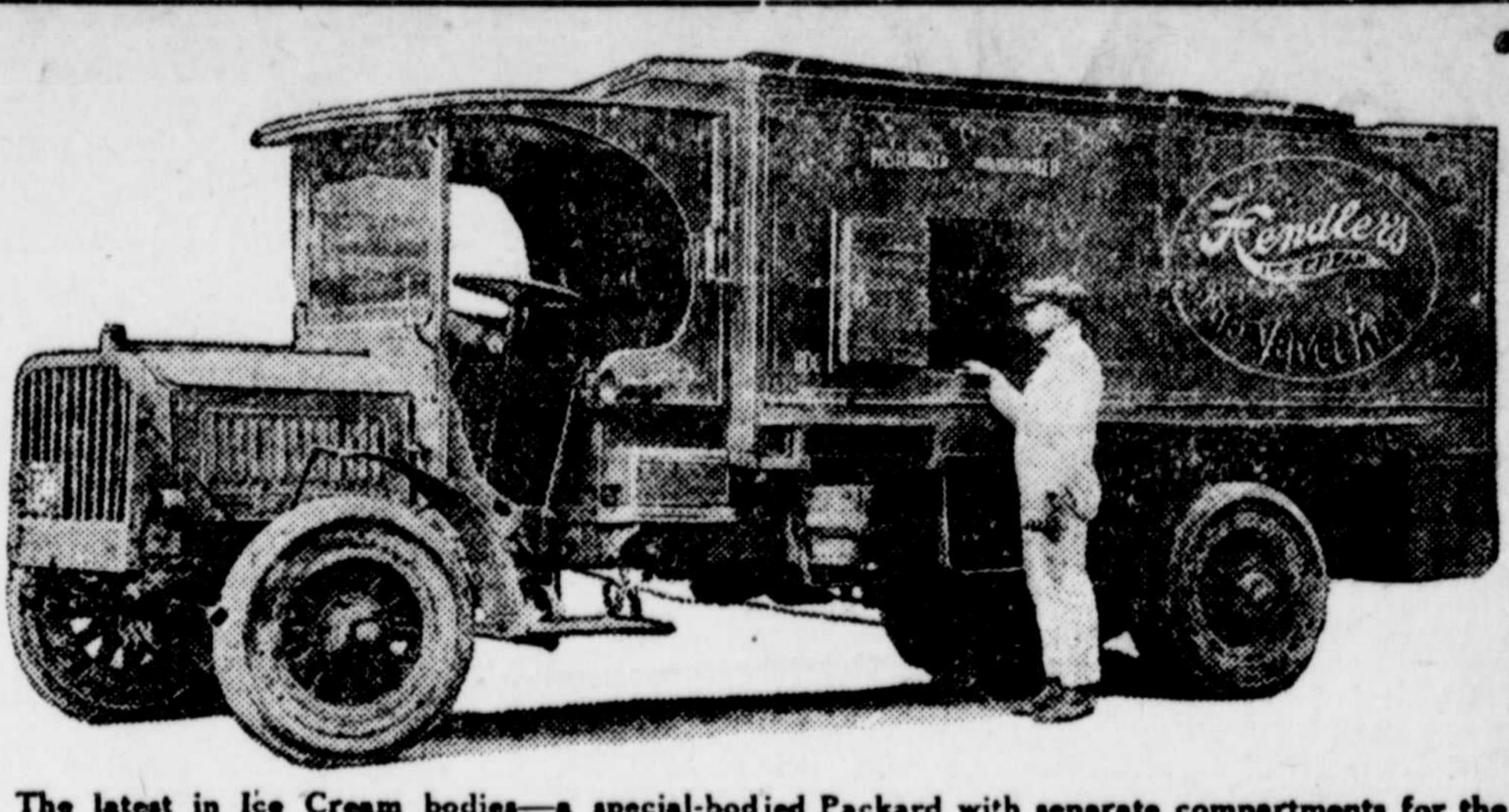
The latest in Ice Cream bodies—a special-bodied Packard with separate compartments for the cream, salt, ice and empty cans. No BRINE to drip and ruin the truck's working parts.
