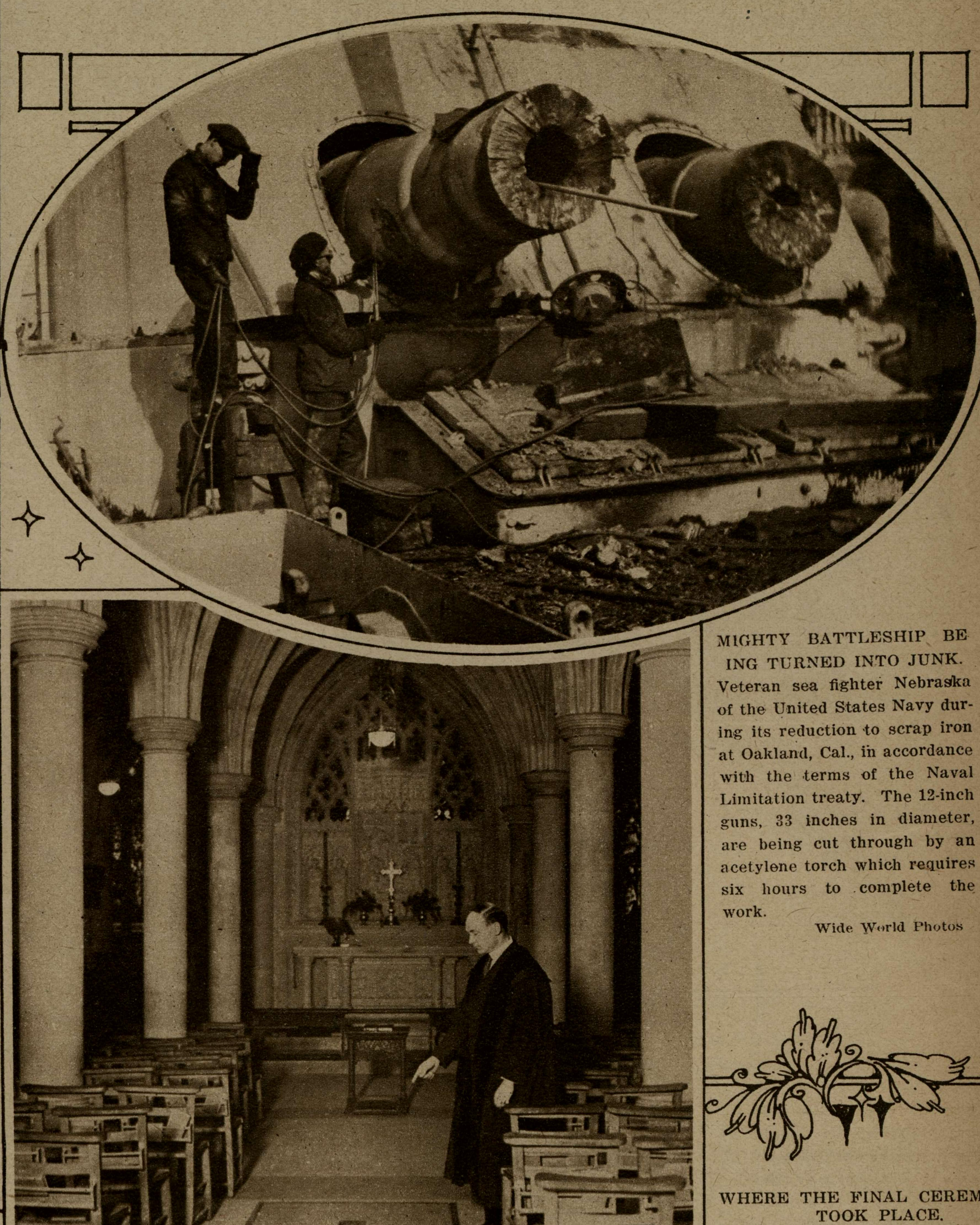
Veteran sea fighter Nebraska of the United States Navy during its reduction to scrap iron at Oakland, Cal., in accordance with the terms of the Naval Limitation treaty. The 12-inch guns, 33 inches in diameter, are being cut through by an acetylene torch which requires six hours to complete the
