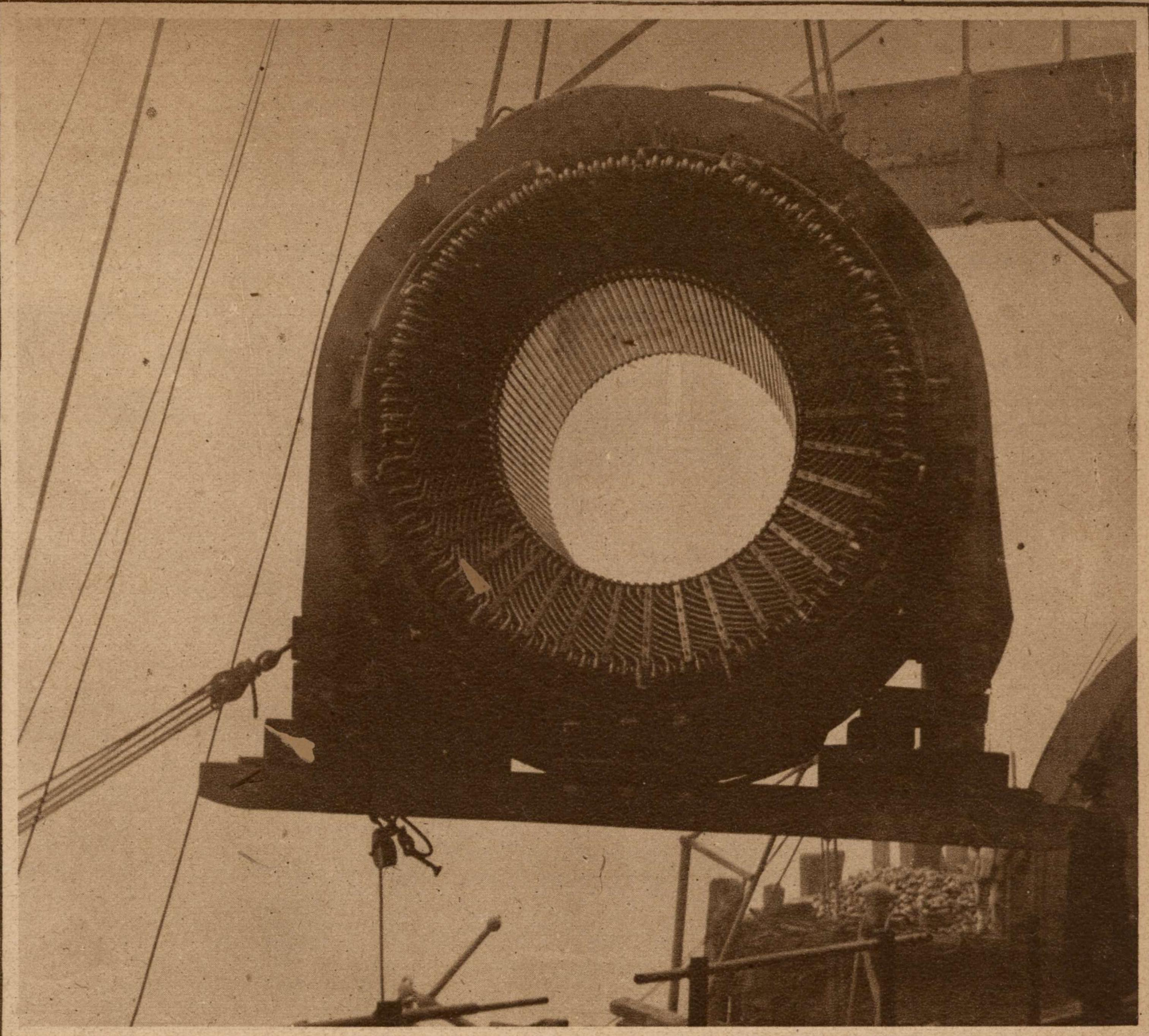
LARGEST ELECTRIC GENERATOR IN THE WORLD.—Turbo-generator of 83,000 horsepower now being constructed by the Edison Company for a power house in Brooklyn, N. Y., at a cost of nearly \$1,000,000. The process of shipment of the gigantic construction, here illustrated, involved the most careful calculation, as it weighs over a quarter of a million pounds.
