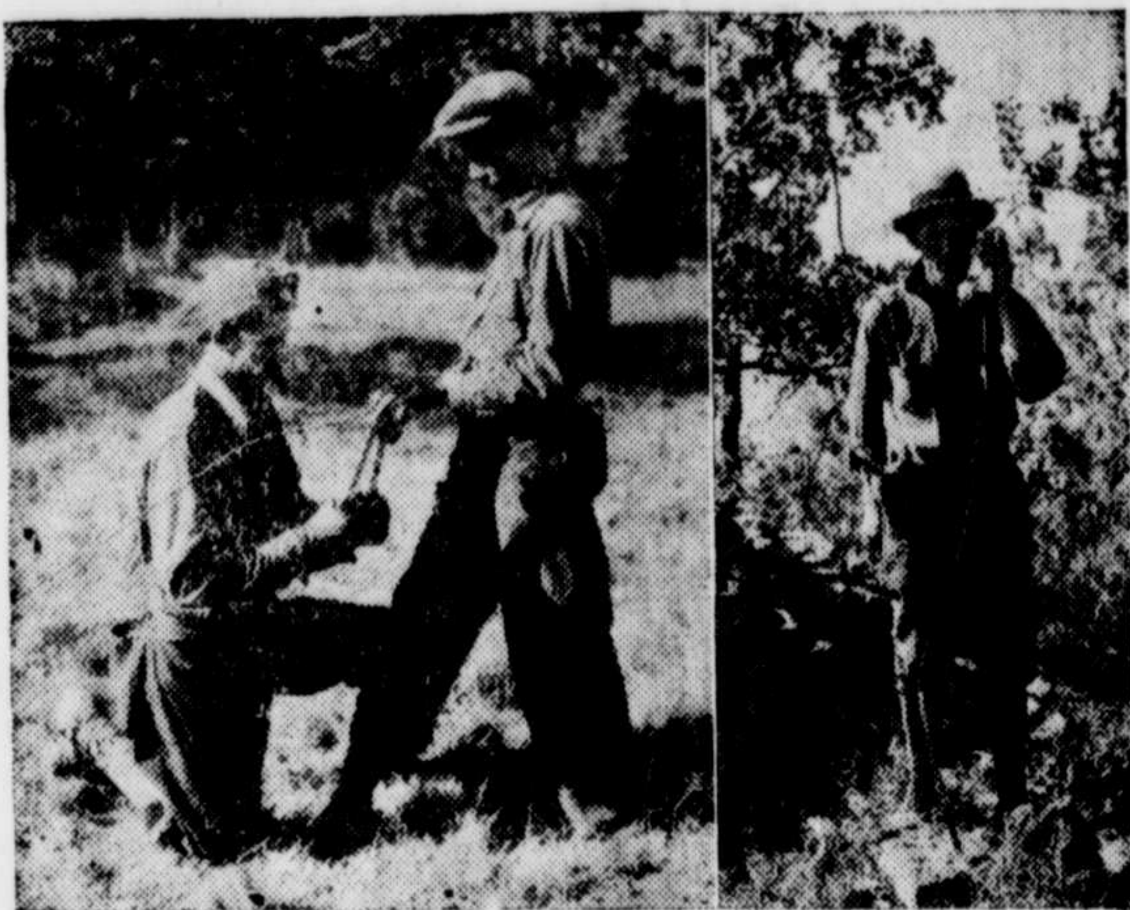
CCC workers splicing a telephone wire in the Monongahela National Forest. (Right) A patrolman with a portable telephone taps in on a forest service line to report a fire just beginning. Forest Service Photos
