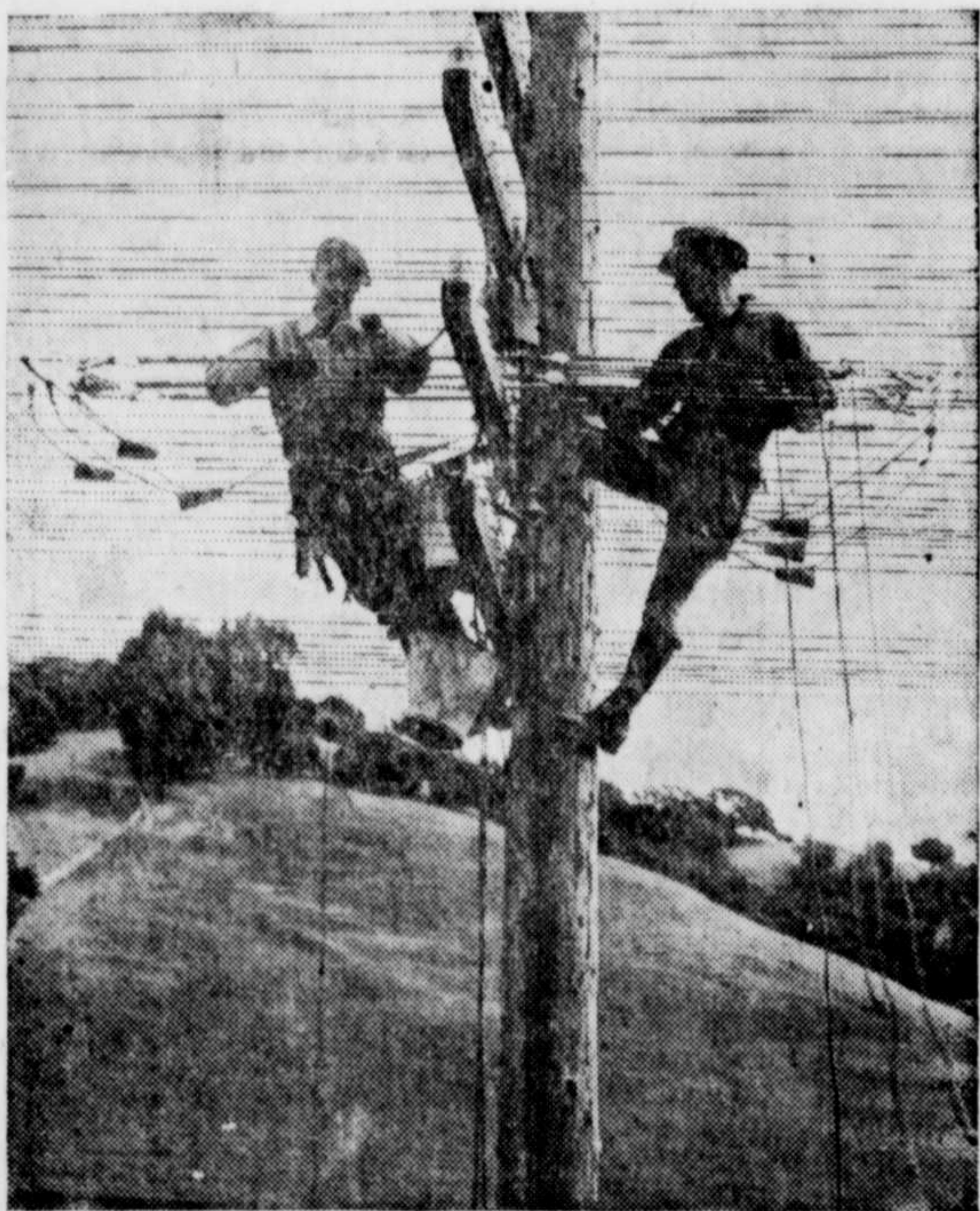
Phantoms—Telephone linemen transposing wires to provide phantom talking circuits.
