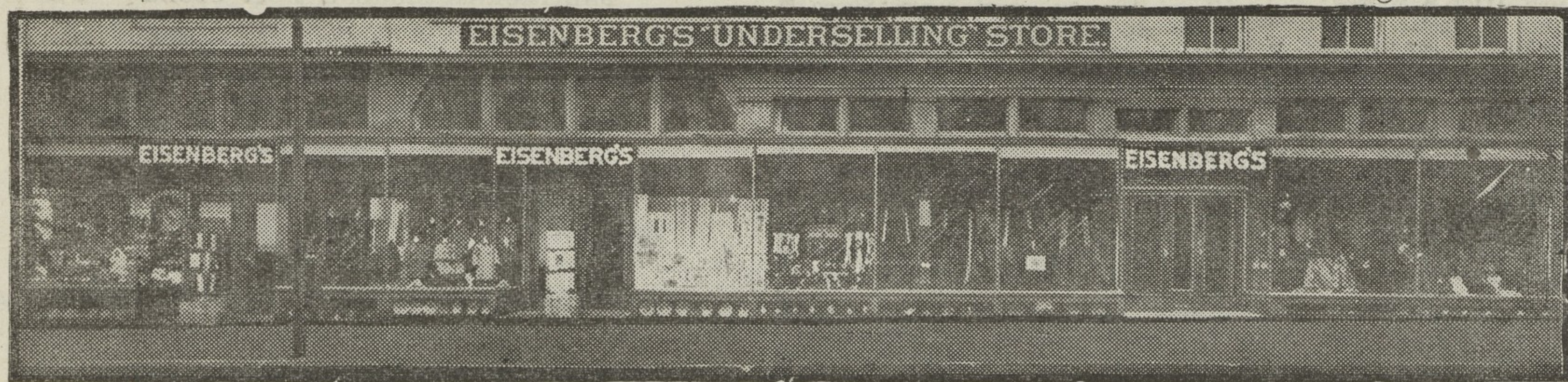
Eisenberg's "Underselling" Store of Baltimore.
